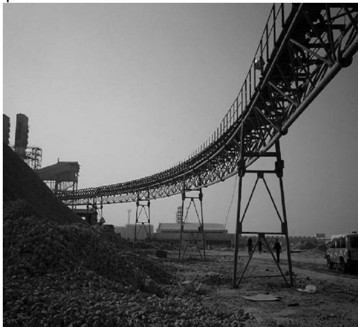
Fig 3: Landing of Coal from the Vessel through conveyor system leading to reduction in Coal Dust Pollution
